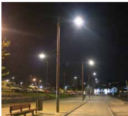
Gloucester Docks public realm light columns
